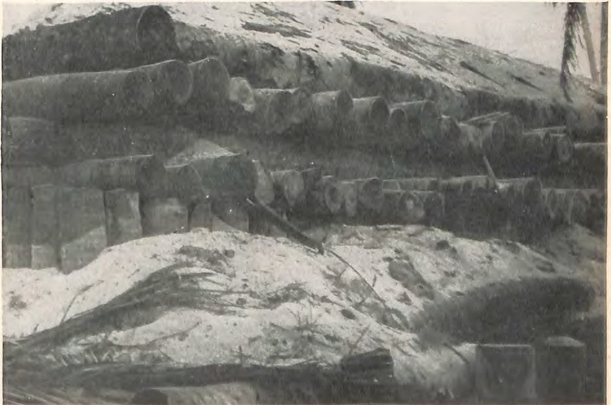
Figure 139. Close-up of typical Japanese bunker.
